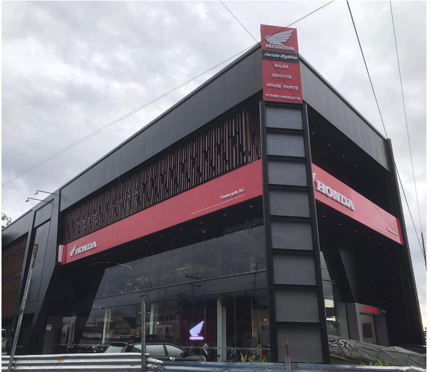
Construction of Honda Showroom exterior and interior.
