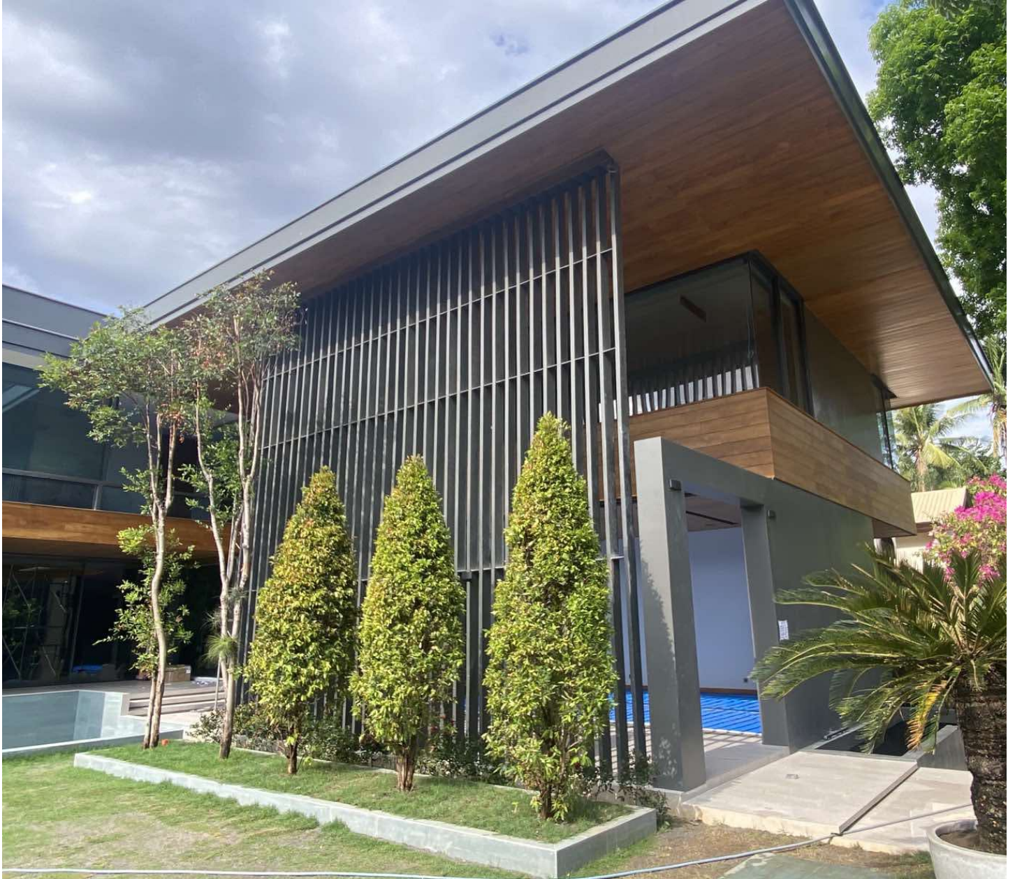
Two storey residential project with basement.
