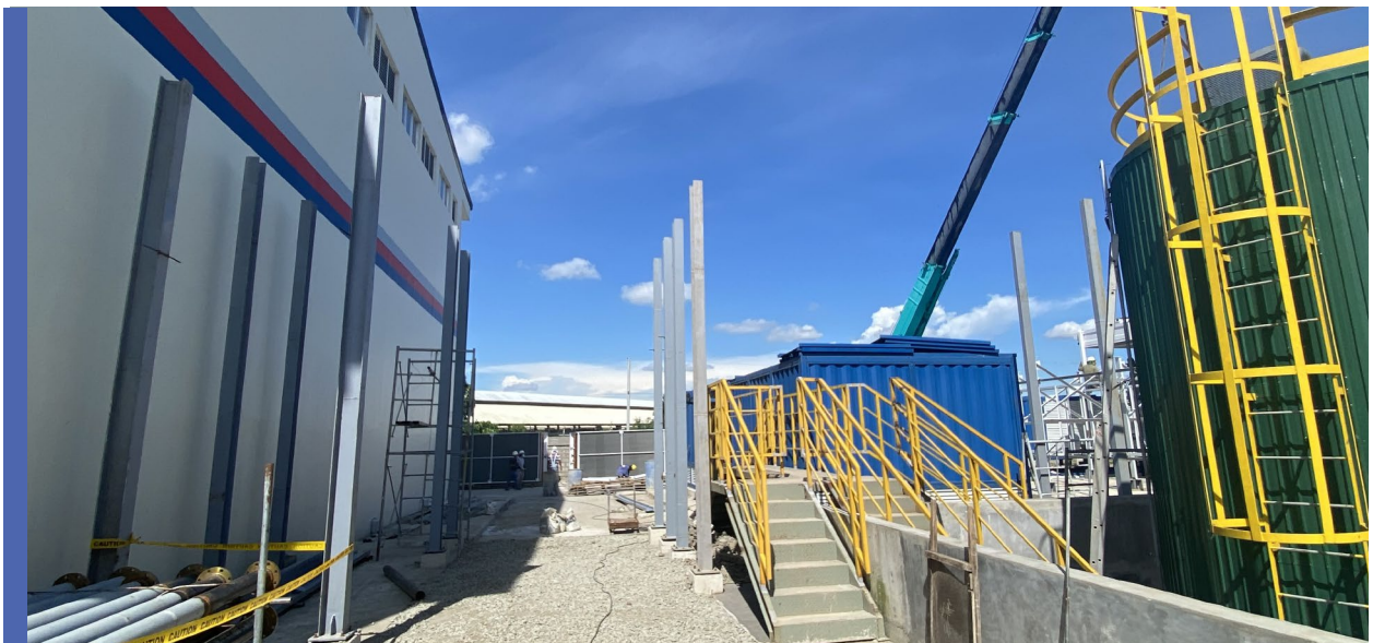
Construction Progress Photos
