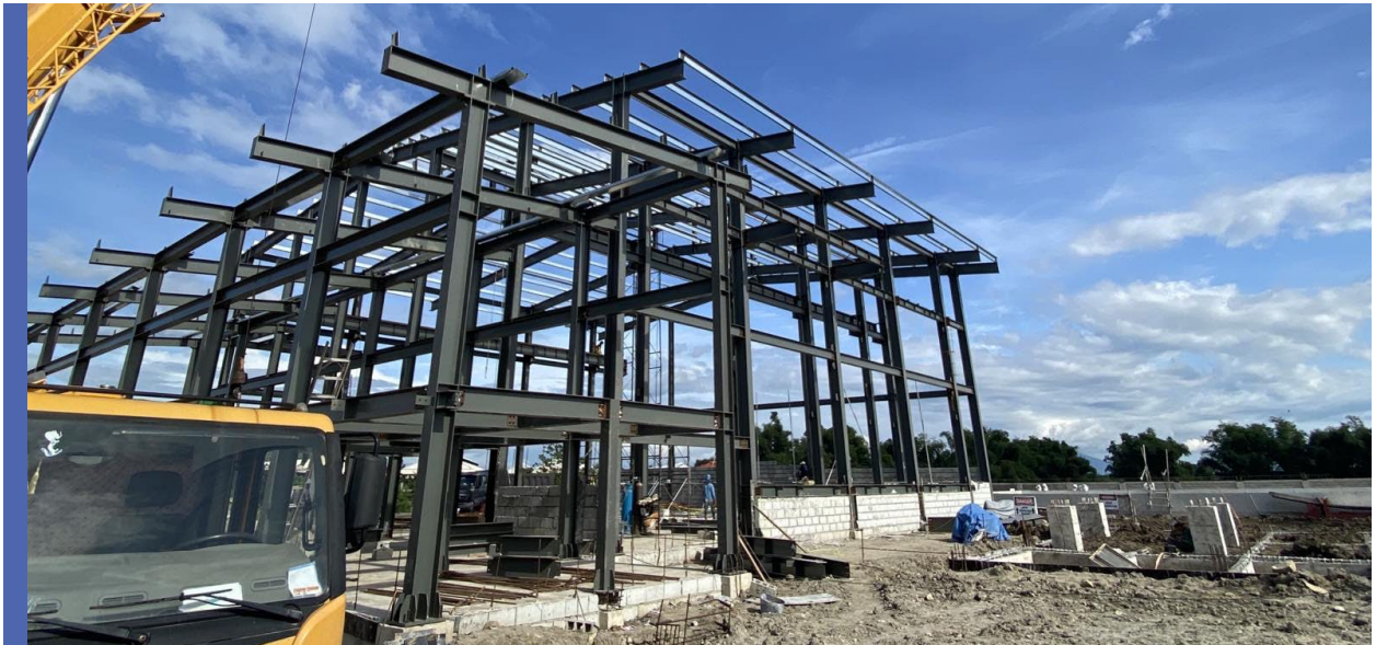
Construction Progress Photos
