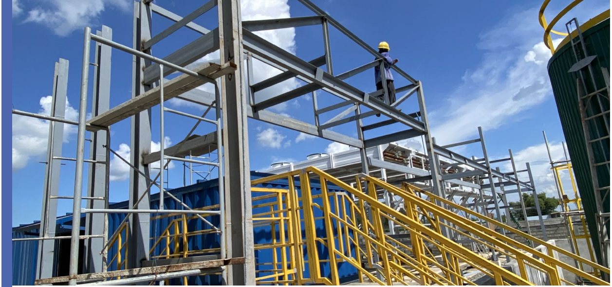
Construction Progress Photos
